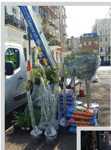
Materials loaded onto the hoist for a fifth floor build
